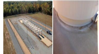
Dominion followed the restart criteria of EPRI NP-6695. The tests and inspections indicated that the earthquake was an EPRI damage intensity of zero; however, the station conservatively followed the inspection and restart guidance for an intensity of one.
